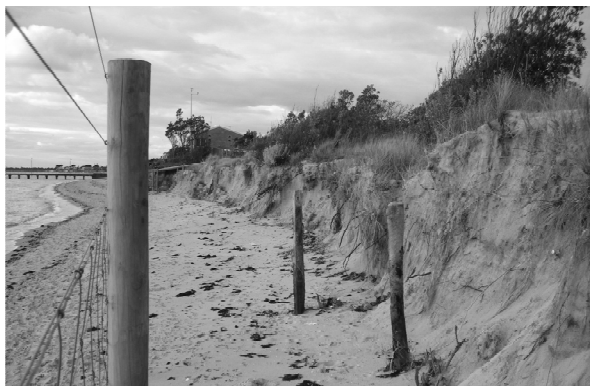
Erosion Damage South of the Coast Guard
